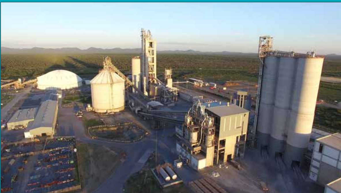
Ohorongo Cement Plant
