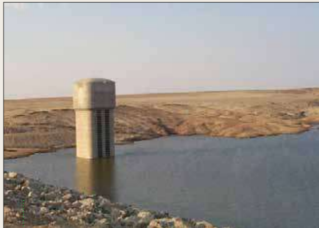
Abstraction tower of the Omdel dam
