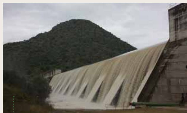
Otjivero dam wall
