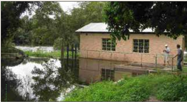
The Andara Power Station
