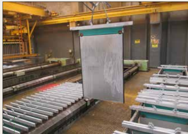
Skorpion Zinc electrolytic plant
