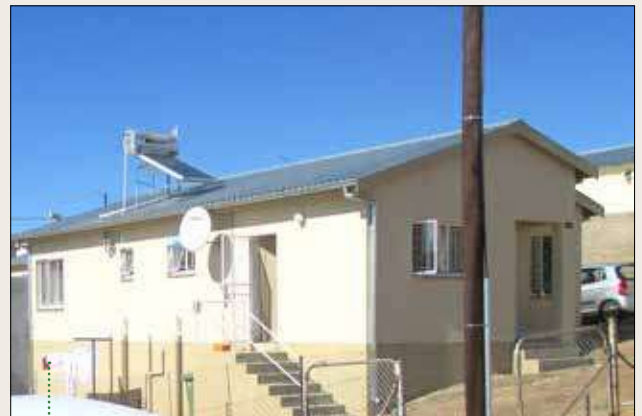
Solar water geysers on the roof of a private home in Windhoek.
