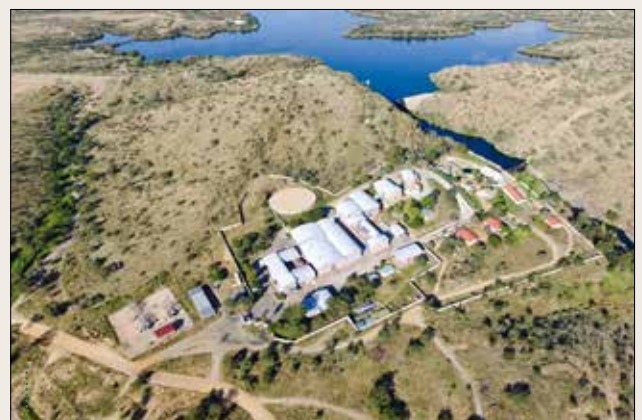
The Windhoek Water Reclamation Plant reclaims potable water from domestic waste water
