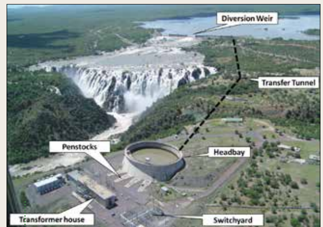
Ruacana Hydropower Station
