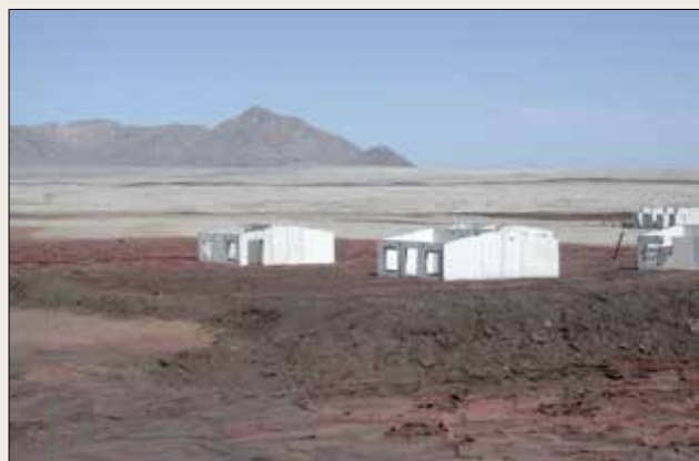
Tailings dam failure
